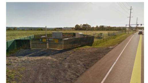
Texas Gas metering station, looking along skew angle of underground 30-inch transmission line (looking west on SR 63; image: GoogleEarth)
