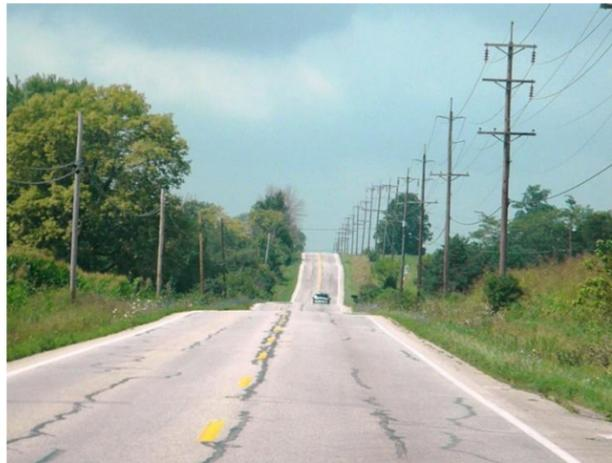
East of SR 741, paved shoulder widths of 1½ to 2 feet are typical (looking westbound near MP 4). Shoulder widths are highly variable throughout the corridor, and variations in travel lane width also occur.
