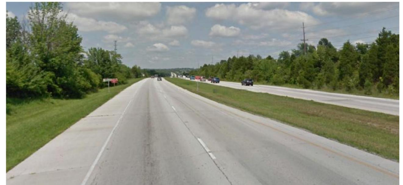
The four-lane section with grass median concept typically uses “open” drainage and provides physical and visual separation of opposing directions of traffic; this example is SR 48 in Warren County, looking north toward Lebanon
