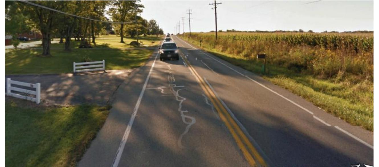
Some sections of existing SR 63 have actual lane widths of significantly less than the 12-foot standard. The Honda compact SUV in this image has an out-to-out width dimension of 5.97 feet. The estimated actual travel lane width at this location is about 10½ feet. (Looking west on SR 63 near MP 6; image: GoogleEarth)
